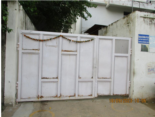
Facility entrance view-min.JPG
